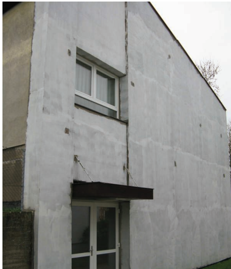
Abb. 1: Photo during the insulation of the outside wall
